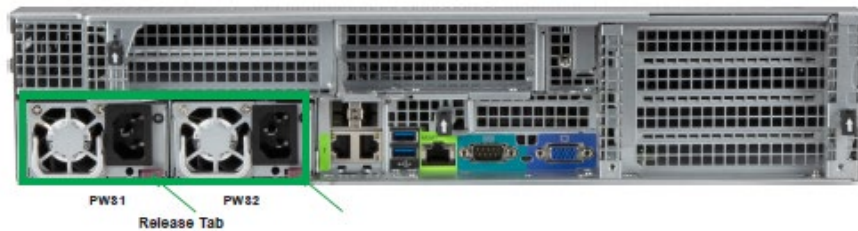
Replacing the Power Supply
