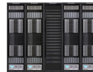
Integrated Rack Solutions
